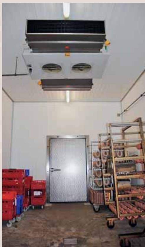
**The AirStream V disinfection module is installed on the ceiling of the production room directly after the evaporator cooler. It reduces the microorganisms at the evaporator cooler and in the ambient air by up to 99 percent.**
