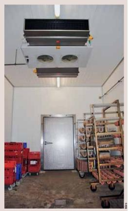
The AirStream V disinfection module is installed on the ceiling of the production room directly after the evaporator cooler. It reduces the microorganisms at the evaporator cooler and in the ambient air by up to 99 percent.
