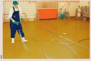
The seamless, water-impermeable Ucrete systems resist intensive cleaning methods with high-pressure, hot steam and aggressive chemicals – they can be cleaned like stainless steel.
